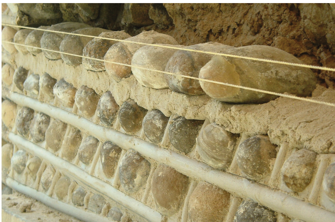
Fig. 12 String lines were used in re-setting the cobble coursing.
