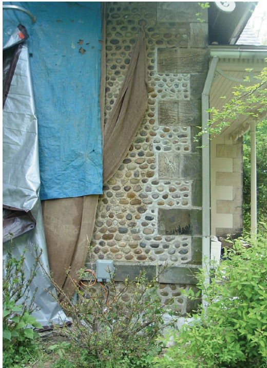
Fig. 8 (right) The south-west corner, with NHL 3 mortar mix.
