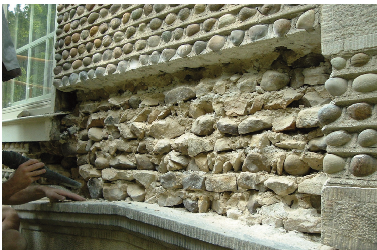
Fig. 11 (below right) Differing mortars in the rubble and cobble skins.
